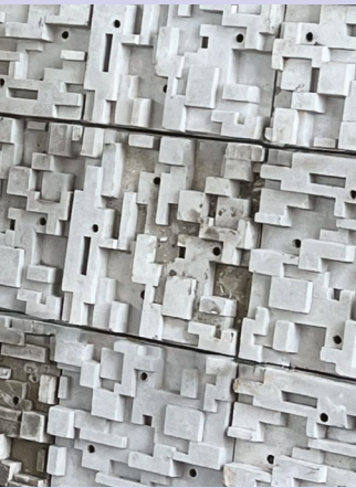
凹凸有致的「生態牆」，可豐富河流生態。 The purposefully uneven “ecological walls” enhance the river’s biodiversity.
